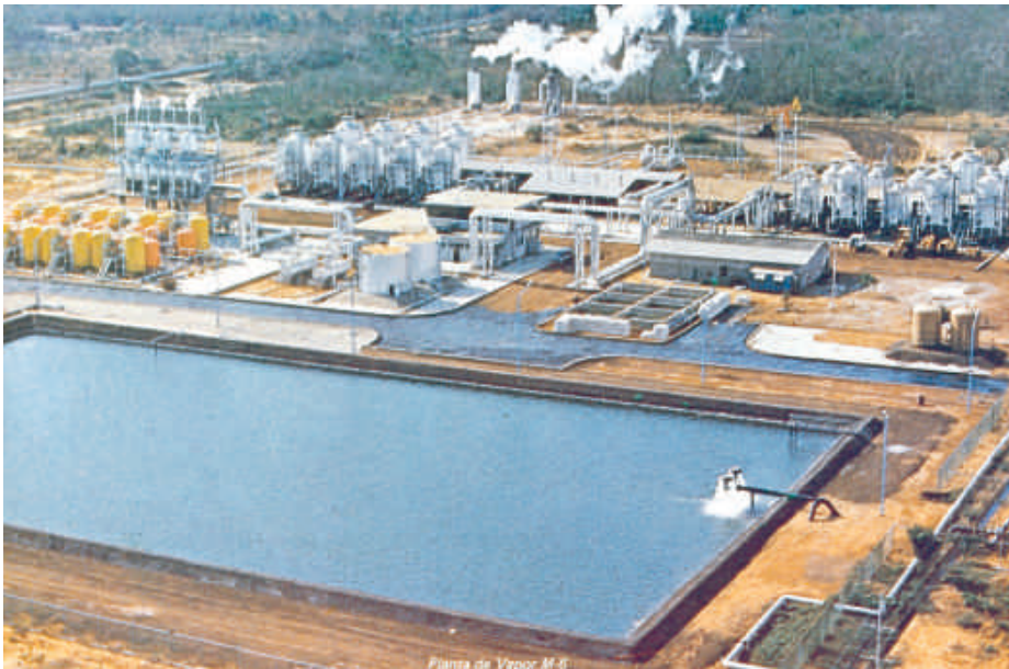
Facility using once through stem generation at EOR site in Venezuela
