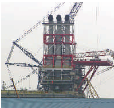
3 nos Water Glycol heaters of 16 MW duty for BP Clair platform phase 1 in the North Sea on a Solar Gas Turbine
